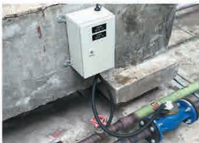
One of the private water meters installed at Wisma Atria to provide early warning of possible pipe leakages
